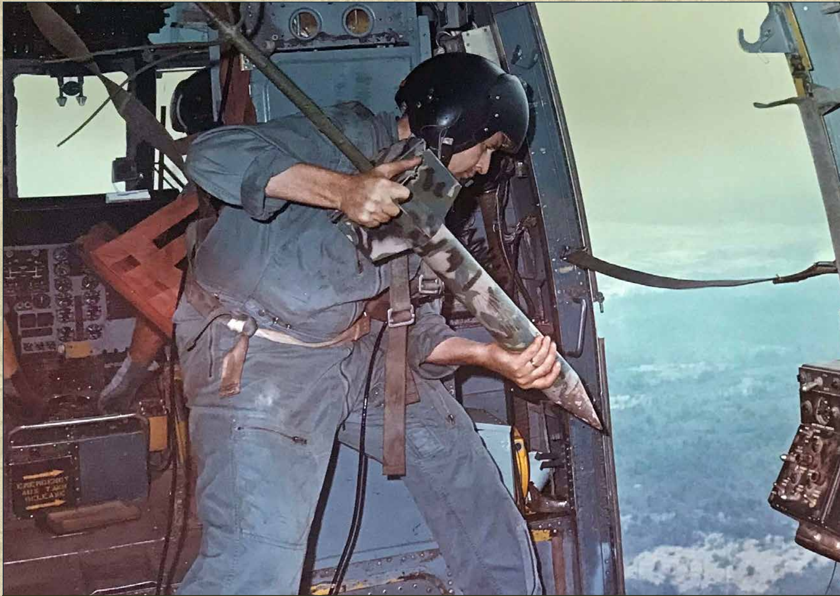
An Airman deploys an Air Delivered Seismic Intrusion Detector from the side door of a CH-3E helicopter. The device senses ground movement and determines whether the source is a person or a vehicle. January 1969. (National Archives)
